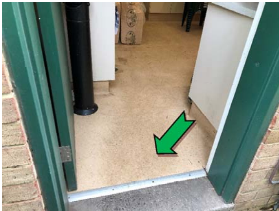
Photo 3. Interior, kitchen, to floor, throughout – non asbestos-containing sheet vinyl.
