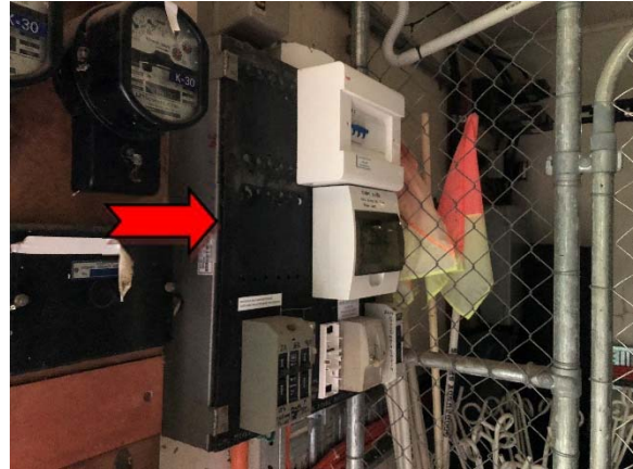
Photo 2. Interior, store room, south-eastern wall – suspected asbestos-containing bituminous backing board.
